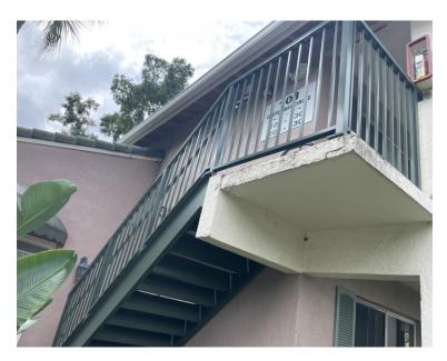
New staircases have recently been installed on some buildings. If painting, the surface will need to be abraded dull. The factory finish should then be primed with BondPlex Acrylic or ProCryl Metal Primer before topcoating.
