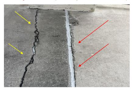
Failing and underperforming sealant should be replaced. Cracks should be routed open and cleaned. Backer rod should be installed in large cracks. Loxon SL1 Self-leveling Urethane should be used in cracks in horizontal concrete. Refer to Crack Repair section (page 15).
