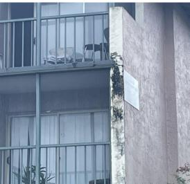
All surfaces to be painted or stained should be thoroughly cleaned to remove dirt, debris, grease, grime, algae, mildew, and any other foreign contaminate. Algae and Mildew should be treated with 1 part bleach to 3 parts water solution, taking care not to adversely affect plant life.
