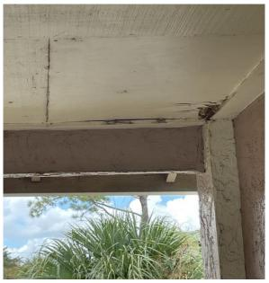
All bare wood should be primed with Problock Latex Primer (B51W620) or Sherwin Williams Exterior Latex Wood Primer (B42W8041). Knotts and tannin bleeding wood may require priming with Oil-based Primer. Rotten and delaminating wood should be replaced. Newly installed wood should be full primed (6-sides) prior to instillation.
