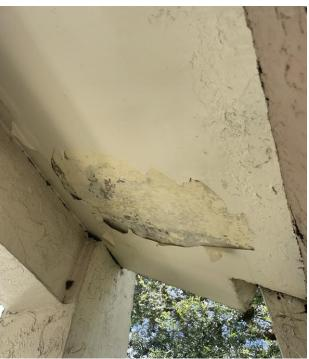
Moisture is causing blisters and adhesion loss of existing ceiling paint. The moisture is most likely gaining acces through the walkways above. Unless moisture is prevented from gaining access, peeling should be expected to continue. Loose and peeling paint should be scraped to a sound surface and the underlying surface should be cleaned free of foreign contaminate. The surface should be primed with Loxon Masonry Primer (LX02 Series) or Problock Latex Primer (B51W620).
